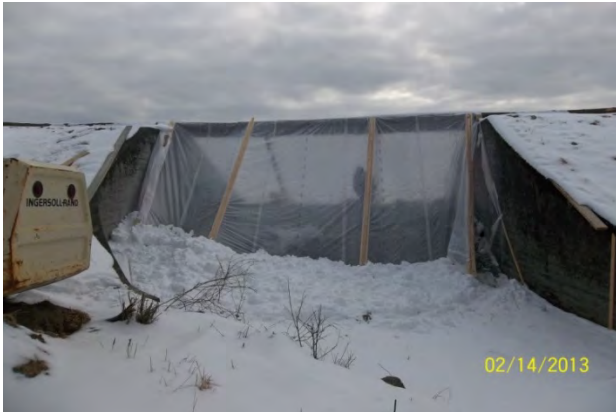
Parker Reservoir Spillway Winter Construction
