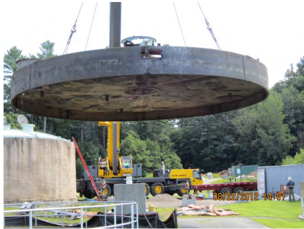
Old Digester Cover Removal
