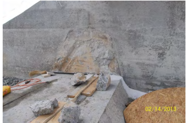
Parker Reservoir Spillway Crest Cut ready for new top
