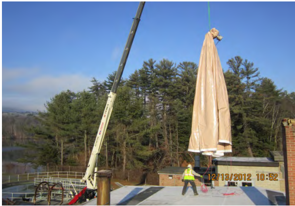
New Gas Holding Cover Installation
