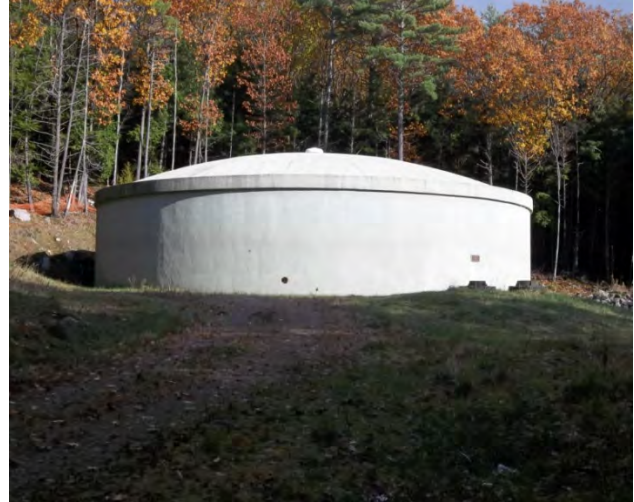
Sand Hill 0.800 Million Gallon Storage Tank
