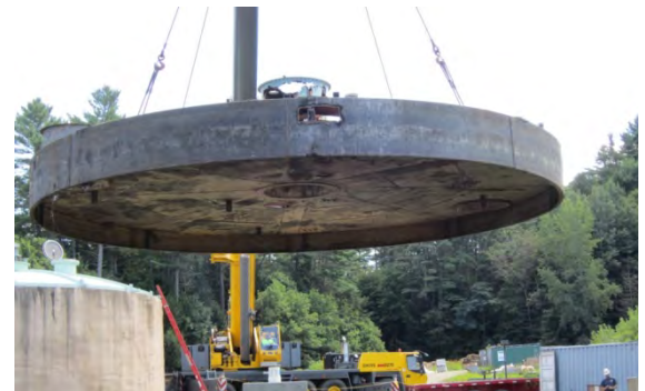
Old Digester Cover Removal
