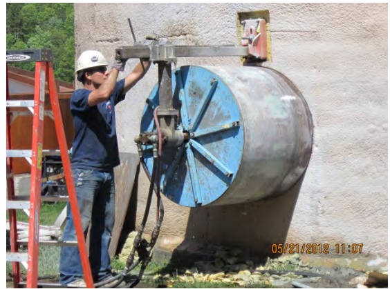
Digester Access Cutting
