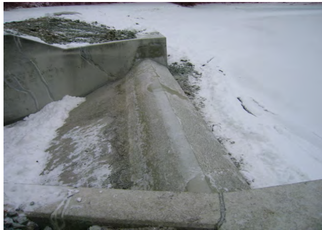
New Lowered Spillway Crest at Fletcher Reservoir
