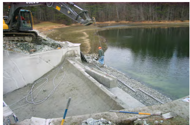
Removing Blocks from Spillway at Fletcher Reservoir
