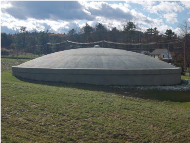
Grasse Road 1.0 Million Gallon Storage Tank
