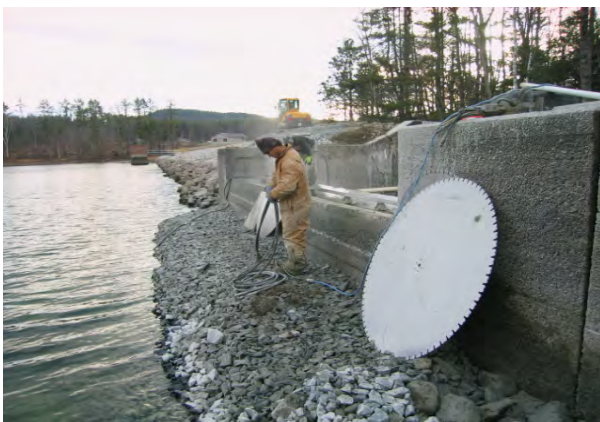
Cutting Spillway at Fletcher Reservoir
