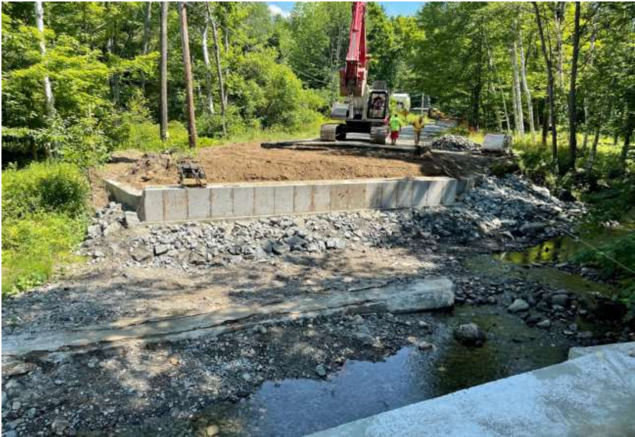
Ruddsboro Road Bridge Replacement
