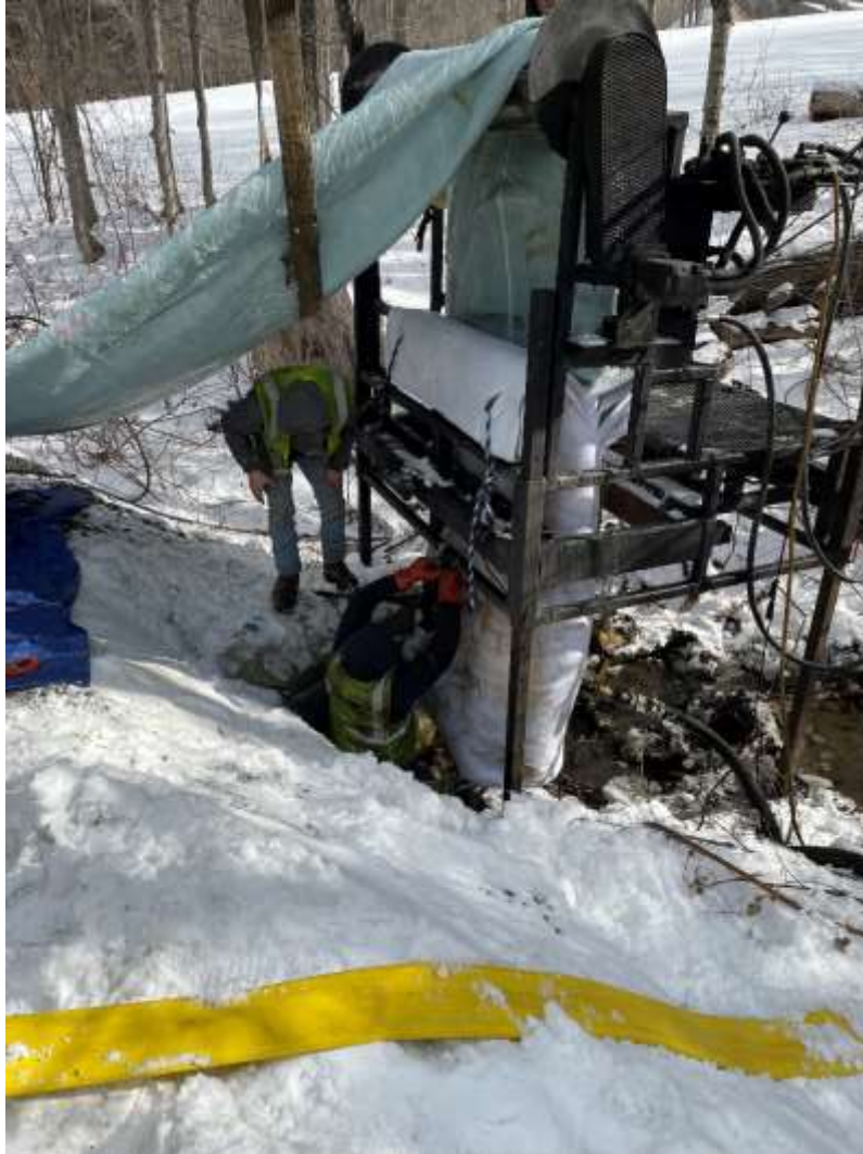
Culvert Sliplining on Stevens Road
