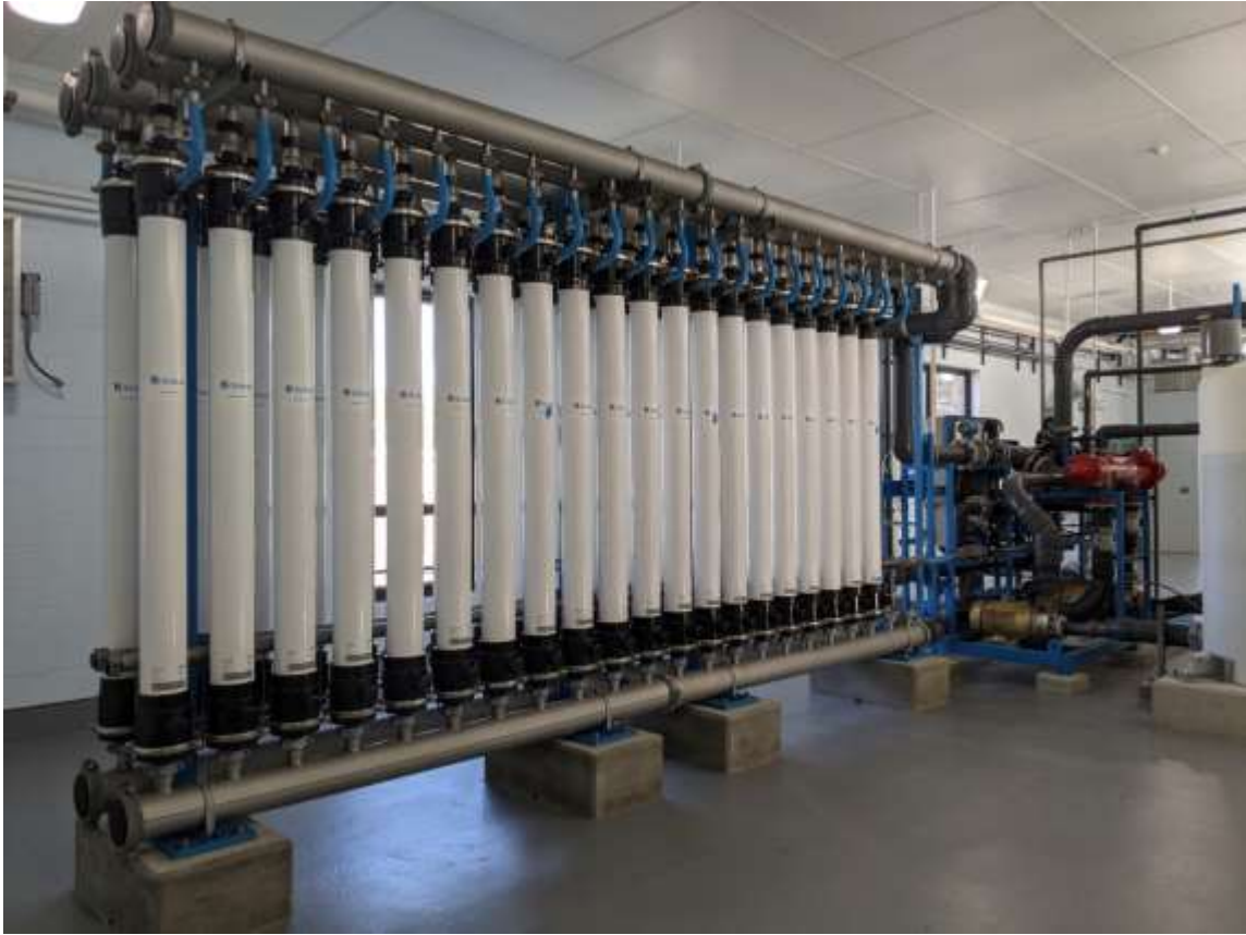
Filtration module replacement at Water Treatment Facility
