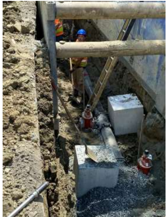
Water Service Line Installation on Hilton Field Lane
