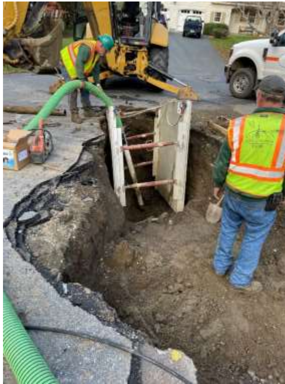
Repairing Water Main Break on Claflin Circle
