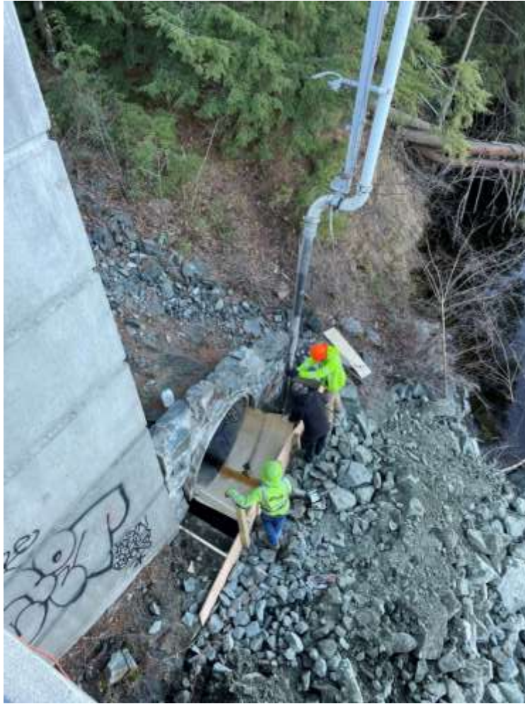
Ledyard Bridge Drain Outlet Repair
