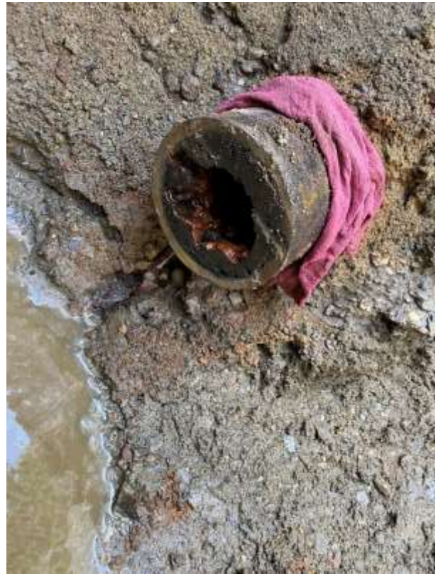
Water Line Replacement on South Main Street
