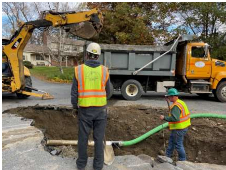
Repairing Water Main Break on Claflin Circle
