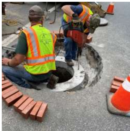
Sewer Manhole Repair on Sand Hill (Lebanon Street)
