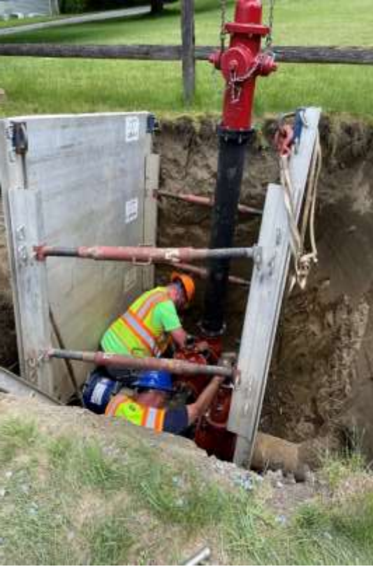
Fire Hydrant Installation on South Main Street
