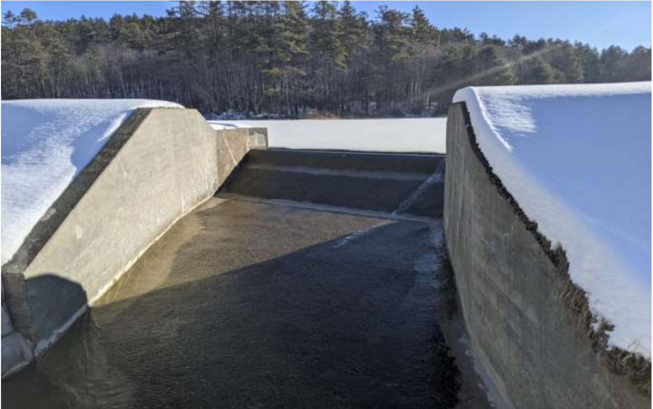
Concrete crack repairs on the Lower Reservoir Spillway
