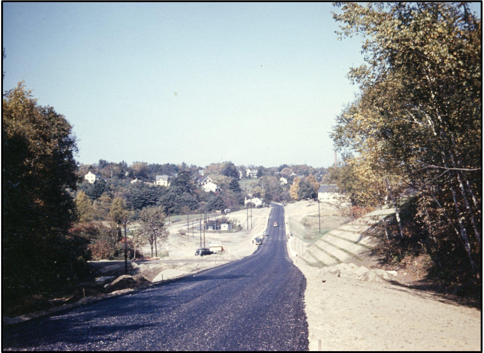
The relocated West Lebanon Road looking north - Summer 1940.
