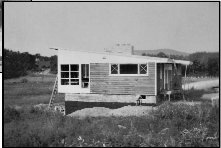
The project to construct 1 Mitchell Lane April to November 1951
