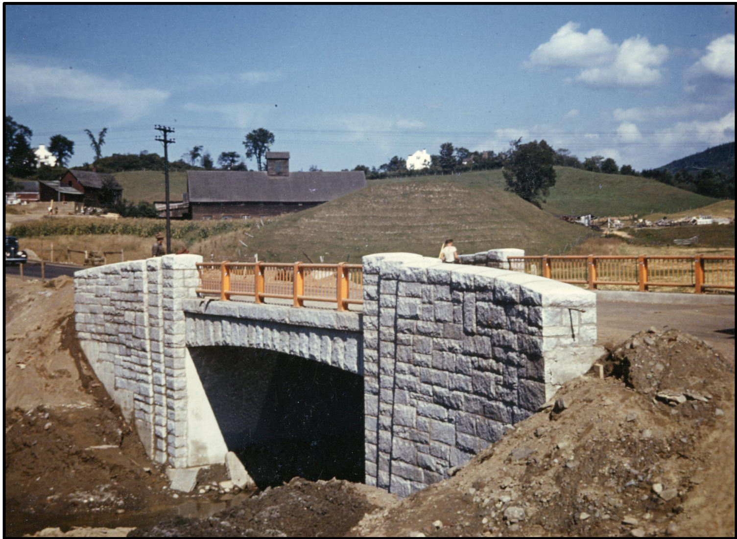
The work to realign the West Lebanon Road included construction of a new Mink Brook bridge and relocating Mink Brook - Summer 1940. The Stone Farm is in the background – looking northeasterly.
